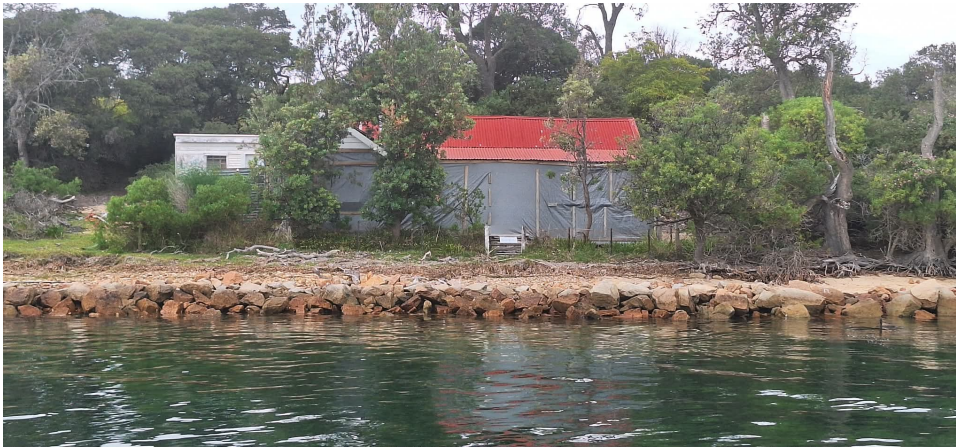
With only the iconic red roof now visible, Schnapper Cottages has been wrapped up to protect the public in December 2025. Another 'nail in the coffin' for this historic dwelling.
