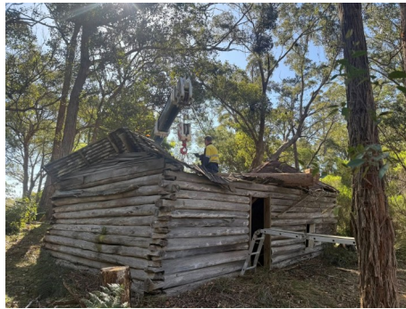
Ready to lift the tree off the roof, Nov 2025
